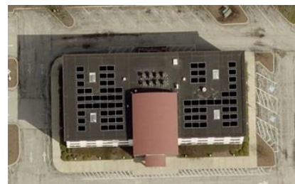
C-PACE loan funded Solar Panels on a roof in Mokena
