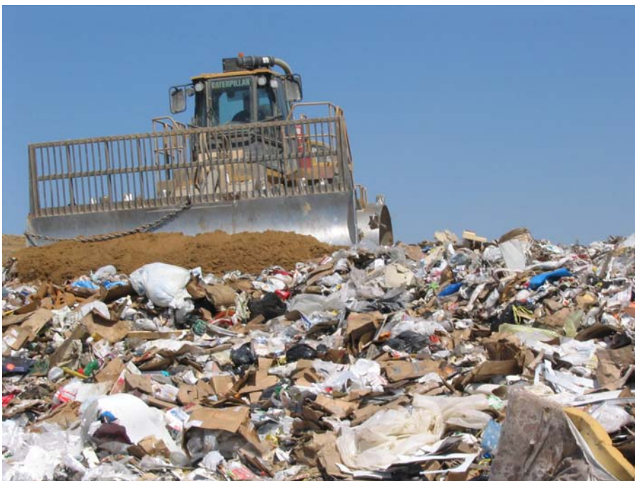
Left – Daily cover being spread over waste at the Prairie View Recycling and Disposal Facility.
