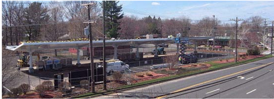
GE's Solar Carport - Rooftop Charging Station, for Electric Vehicles – April, 2011
