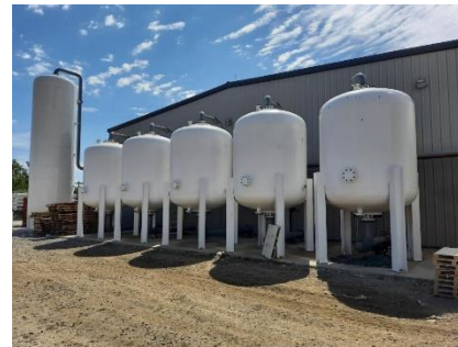
Construction continues on Will County's RNG Plant
